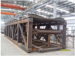
Highkelly steel manufacturing facility
