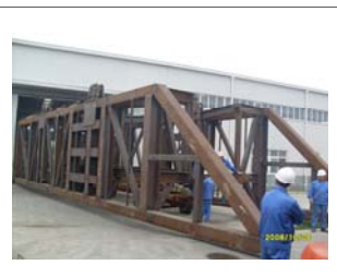
Highkelly staff preparing a substructure for paint.
